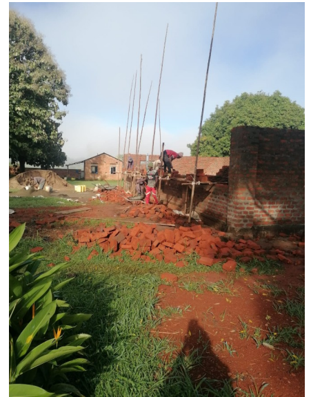
Working on the chapel
