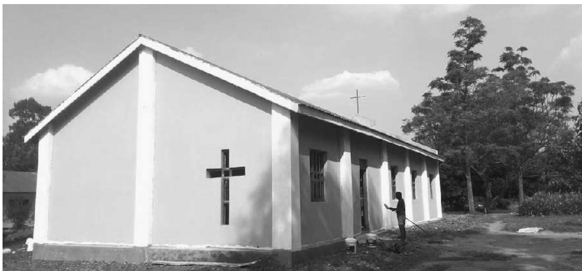
The new chapel, built by willing volunteers.
